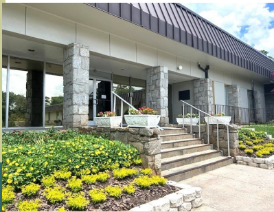
Our exterior was refreshed with gray paint, new soffits, and more.
